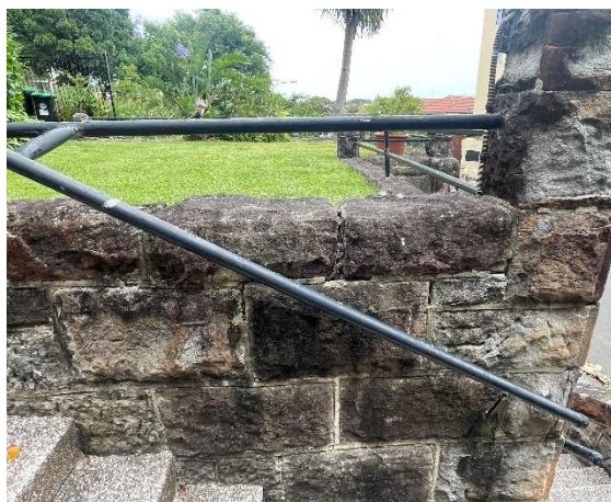
Photograph-6: Loss of mortar/cracking in retaining wall. View looking south.
