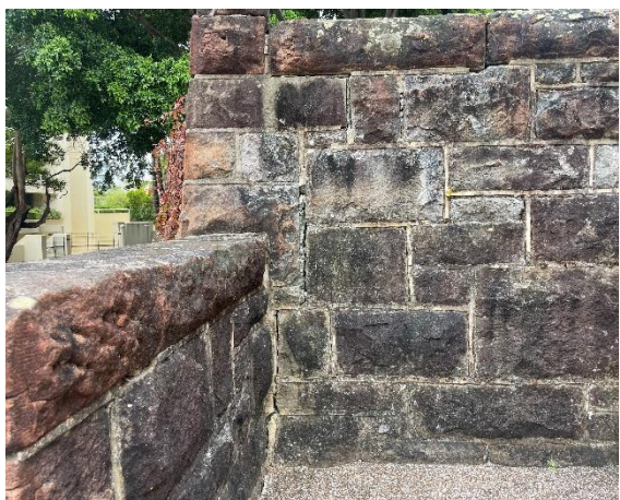
Photograph-5: Loss of mortar/cracking in retaining wall. View looking north.
